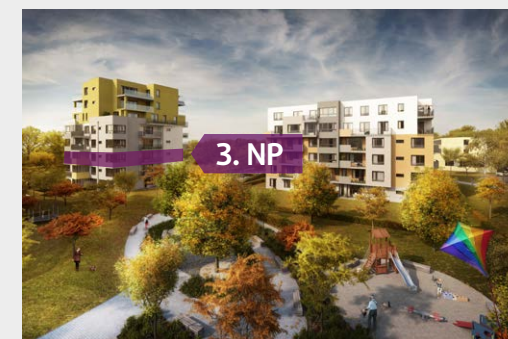
Pohled na dům / Building View
