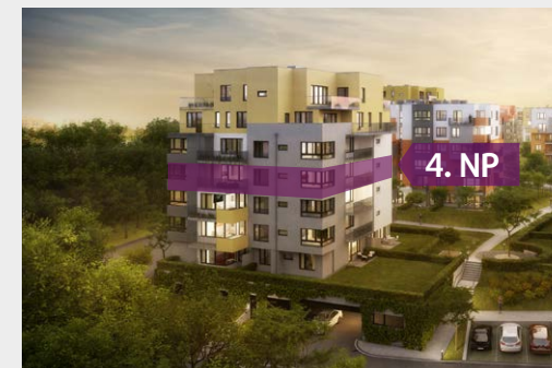
Pohled na dům / Building View
